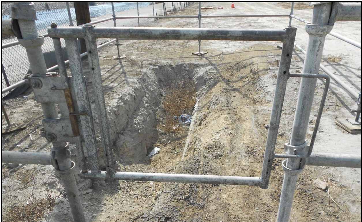
Photo 4. Trenching section for new pipeline. Segment: 1
