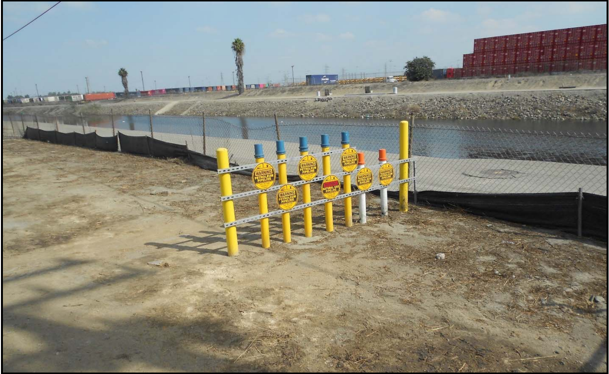
Photo 7. View of pipeline markers along pipeline corridor.
