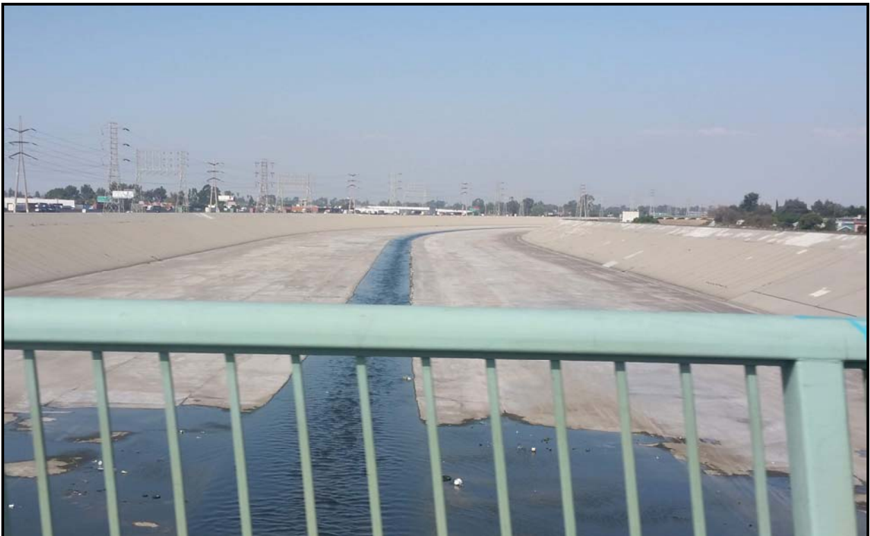
Photo 10. The Los Angeles River at the pipeline crossing. Segment: 5.
