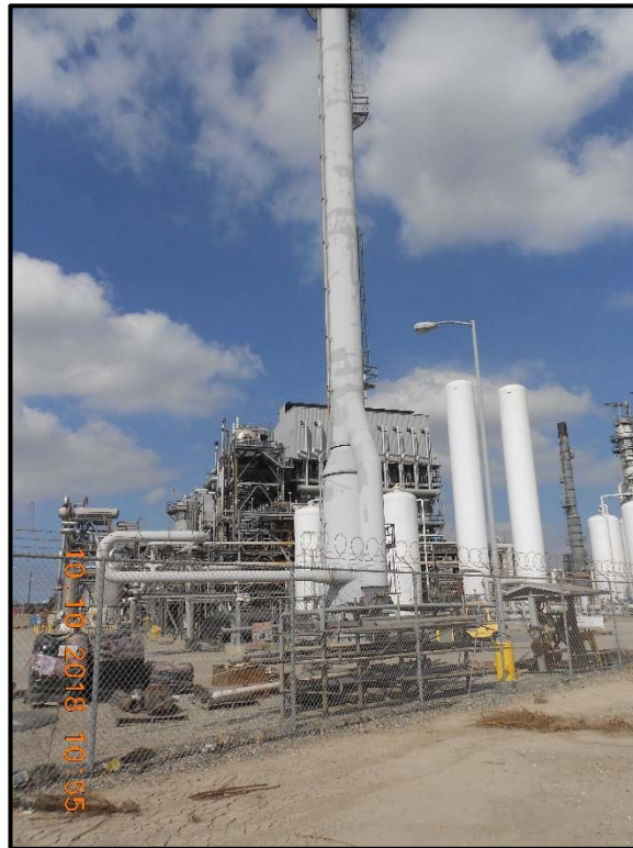
Photo 2. Air Products Hydrogen plant in Carson. Segment:1
