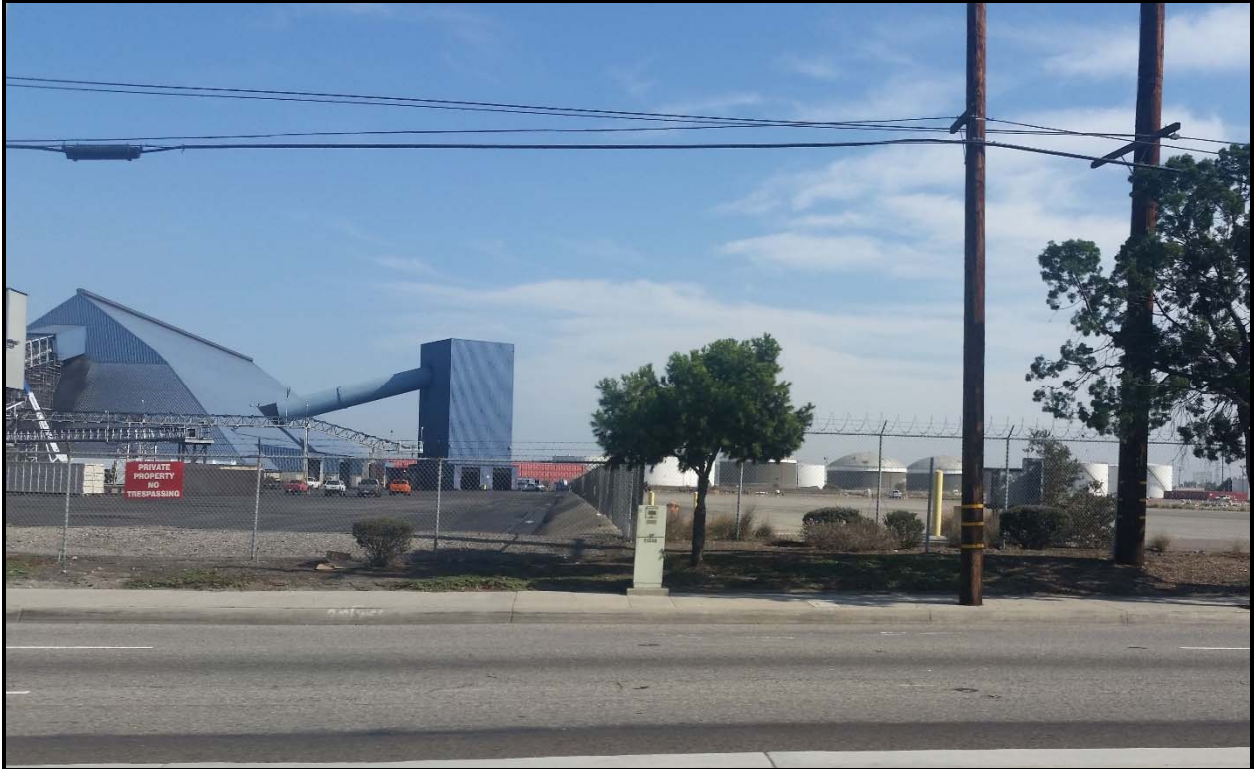
Photo 5. Petroleum coke facility along pipeline route.
