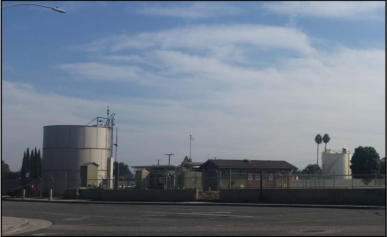
Photo 7. Industrial area along the pipeline route on Alameda Street. Segment: 3
