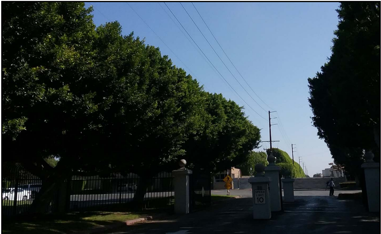
Photo 18. Entrance gate to the Paramount Refinery. Segment: 10
