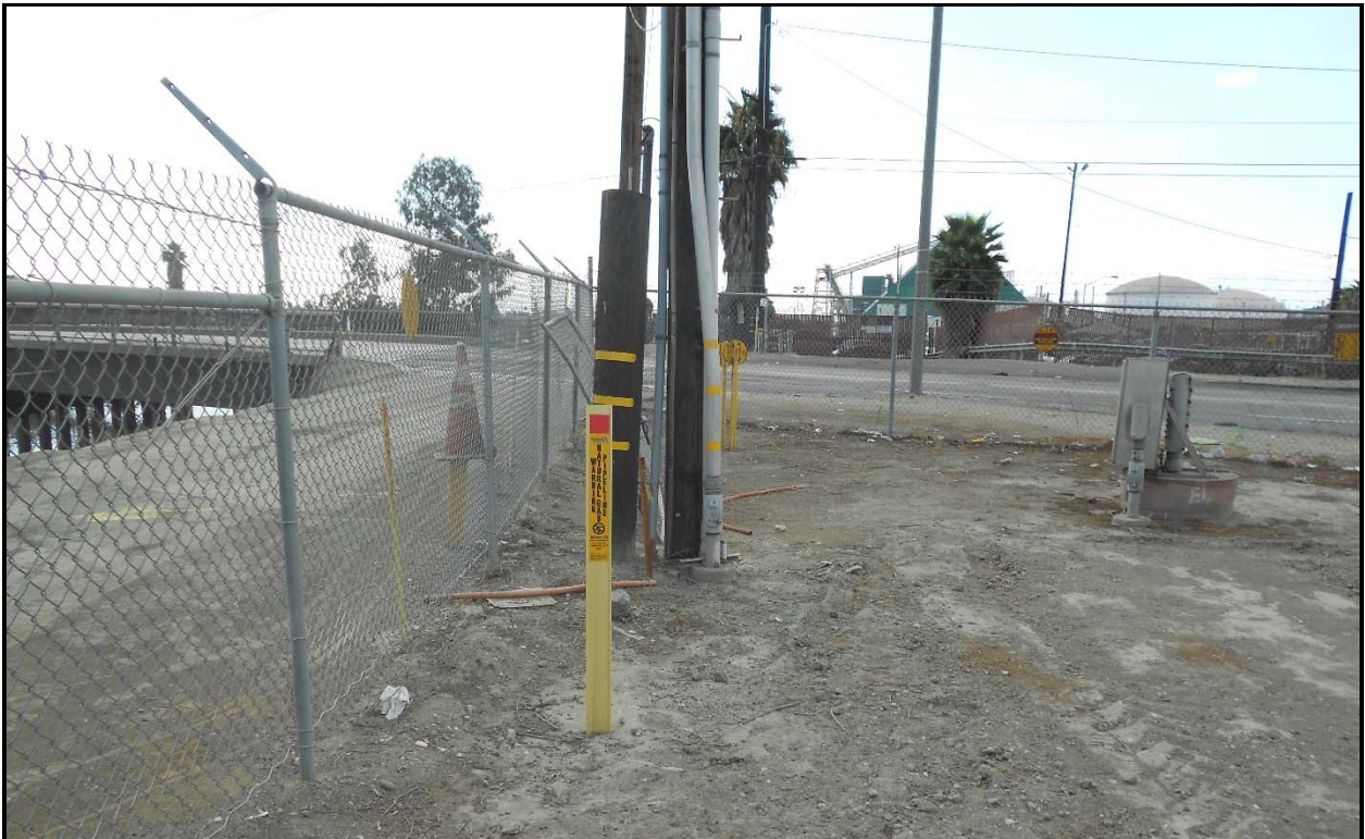
Photo 8. View of End of pipeline corridor area at Sepulveda Boulevard.
