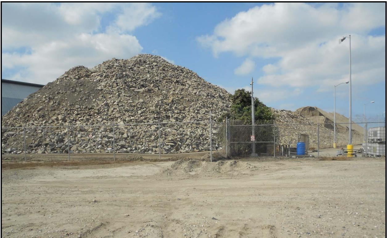
Photo 6. View of Concrete Recycling Facility west of pipeline corridor.
