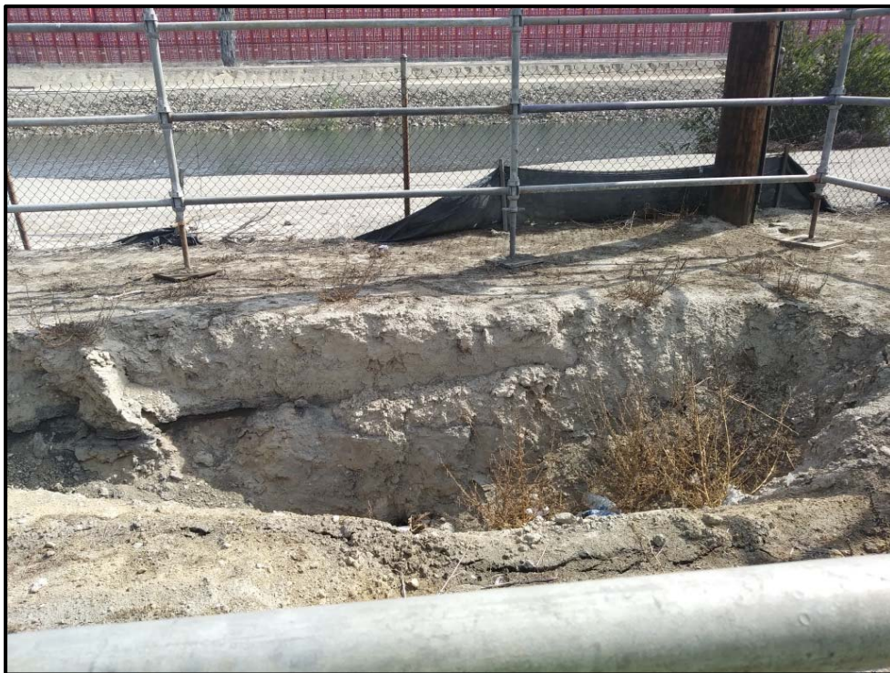
Figure 5-4. Previously excavated trench along the north-south segment.
