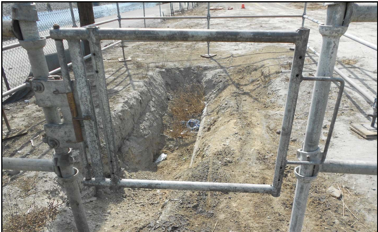
Photo 4. Trenching section for new pipeline. Segment: 1
