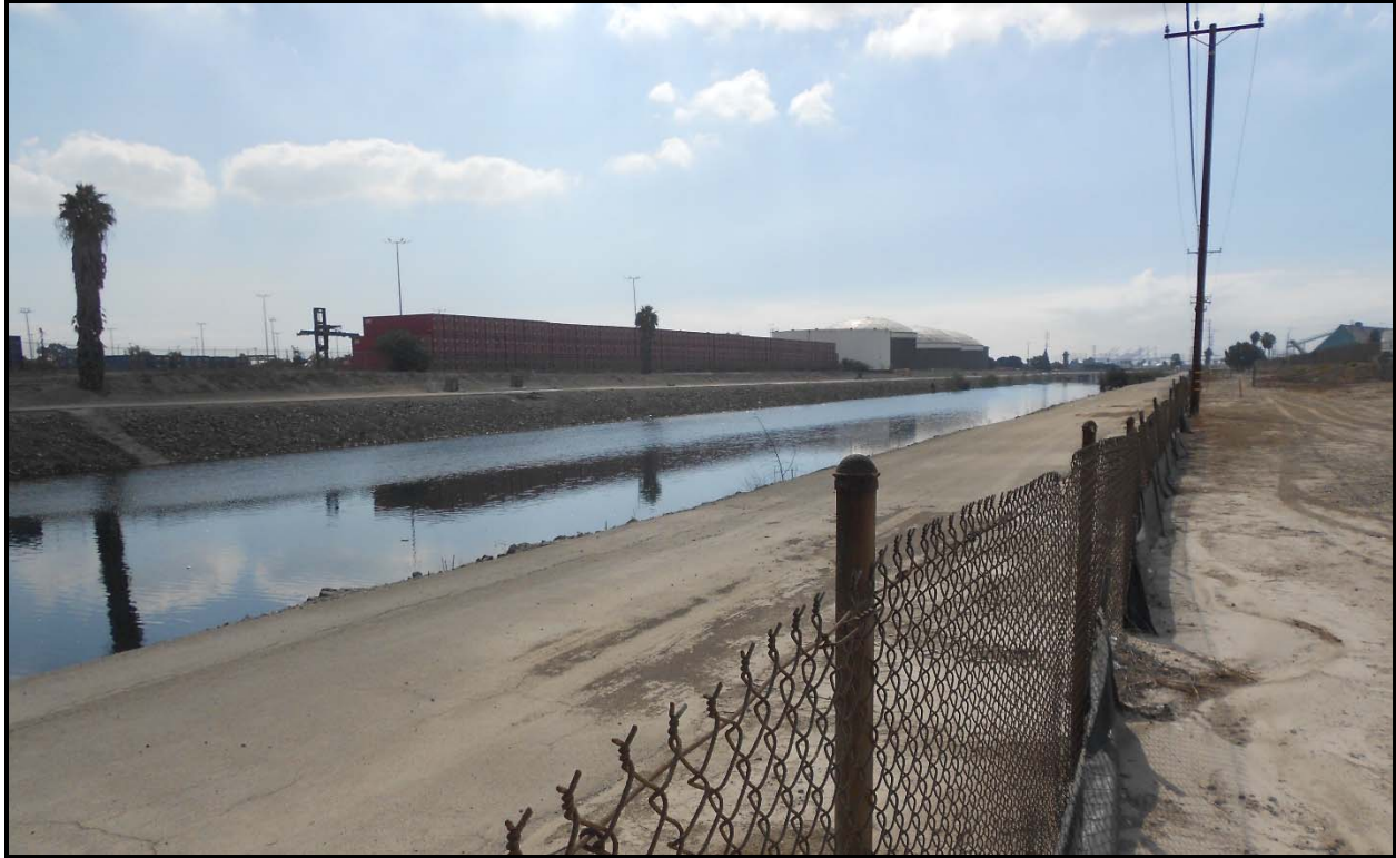
Photo 3. Dominguez Channel as bordered new pipeline at the Carson Facility. Segment: 1
